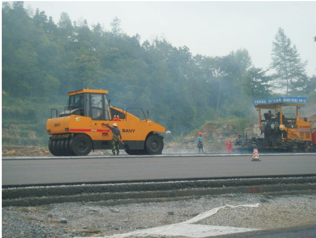
SPR360 is under construction on 19 section of Jicha expressway in 2011
